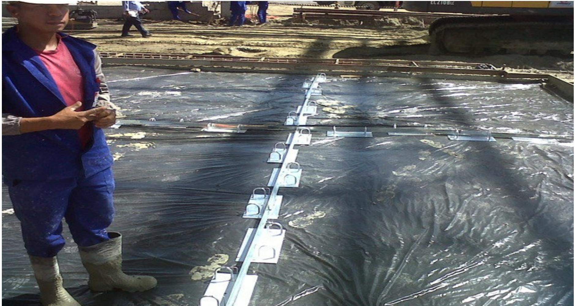
Example of load transmission steel plates over plastic film
