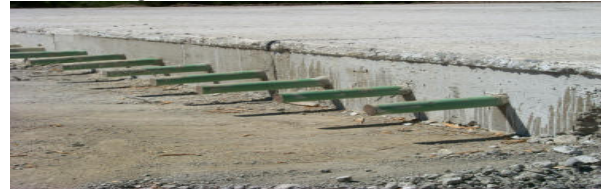
Steel Load Transfer Bars (DOWEL BARS)
